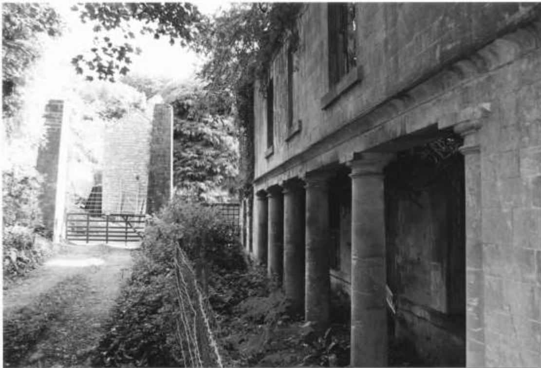
The front entrance to the offices of De Montalt Mill. The two 'pylons' at the far end supported the 'launder' or duct carrying the water from the millpond (left) to the top of the wheel which stood against the side of the building.
